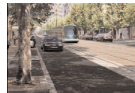
Avenue Gorbella MOER Tram
